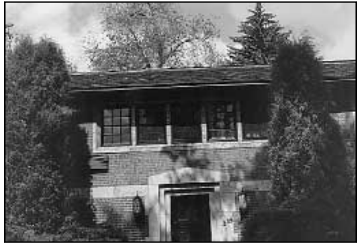
Typically windows of historic houses are vertical. Groupings of windows such as this create a horizontal band.
