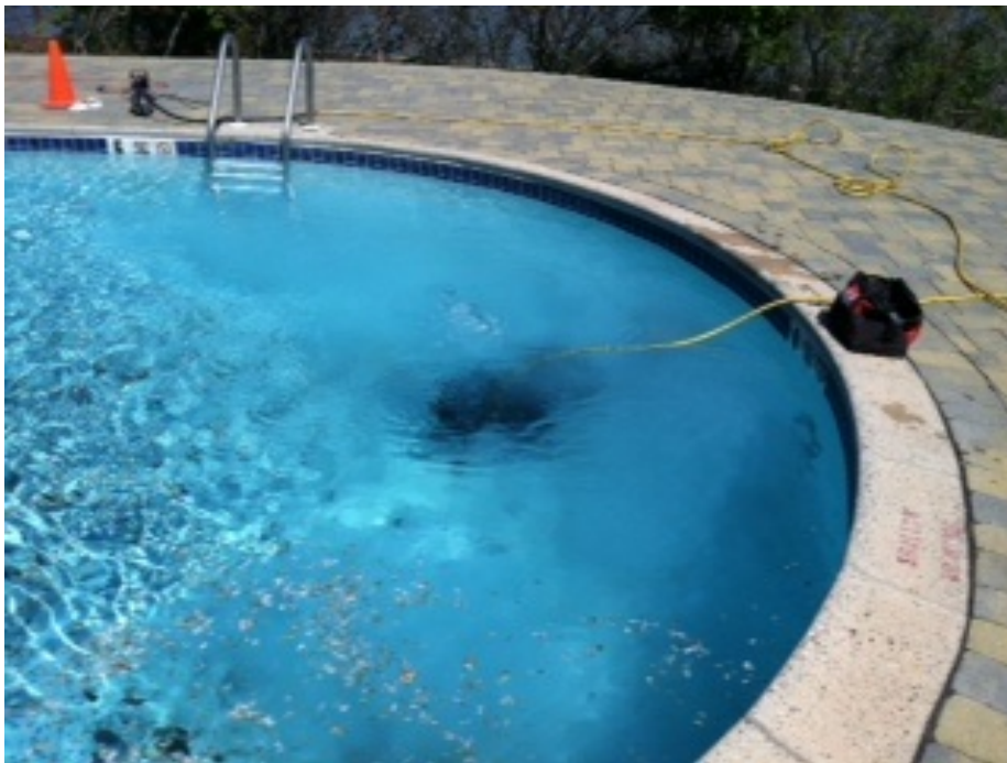
Scuba diver testing the main drains
