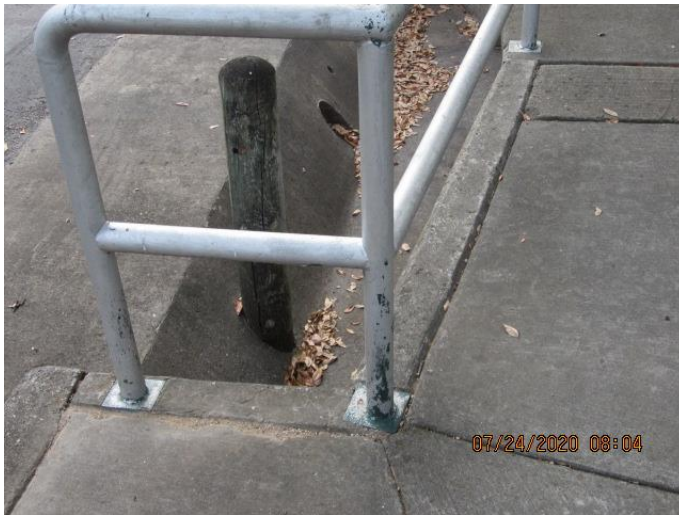
West Park Culvert - July 2020
