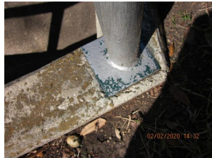
East Park Culvert – Feb 2020
