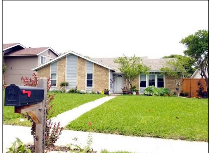
SOUTH – BRADLEY & HELMICH LEQUIRE, 3113 NOBLE LANE
